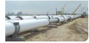
The polyisocyanurate injection systems for seamless LNG pipes' insulation before installation on site. Thanks to the fast yet precise application process under indoor controlled conditions, SPINPIPE ensures maximum guality control, insulating shell's repeatability and operators' safety. Low environmental impact (ODP = 0, GWP < 1) and full compliance to strictest cryogenic specifications make SPINPIPE the optimal solution to improve efficiency and logistics of major LNG projects.
